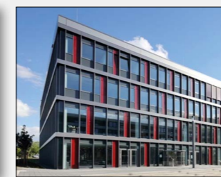
Parapet / façade elements
